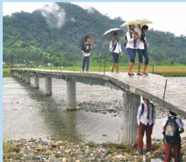
Student crossing the newly built trail bridge
